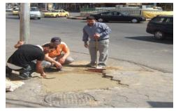
Figure 16. Add an earlier ramp to the pavement (on the left) and adjust the slope of the pavement after its collapse (on the right).
